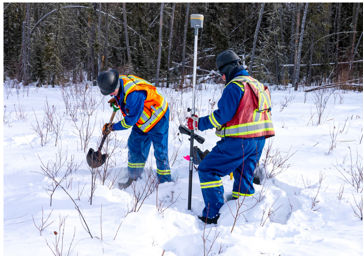
Surveying for Pathways transportation line in existing rights-of-way
