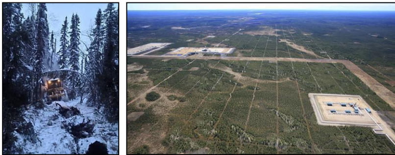
Figure 2 - (left) Equipment clearing corridors for low impact seismic exploration and (right) an aerial view of 2D seismic exploration.
