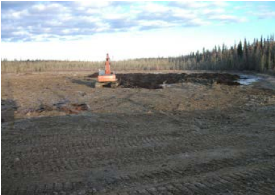
Mounding of remaining fill, producing mixed surface substrate.
