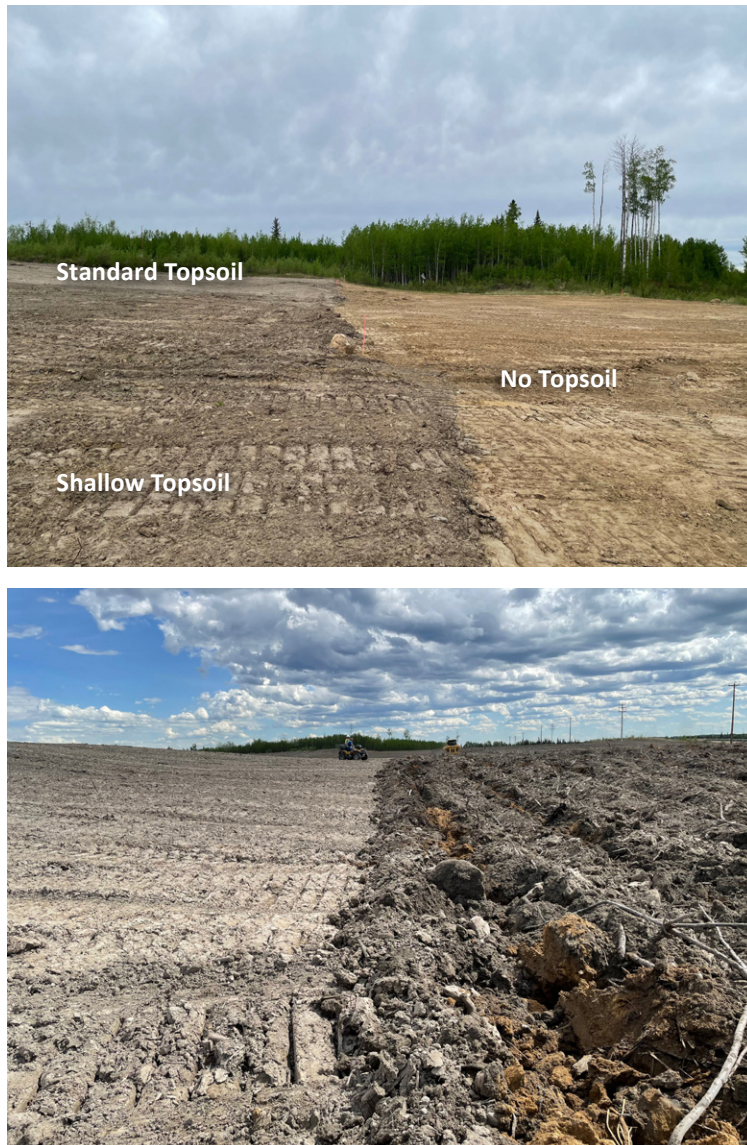
Figure 2: Images from June 2021. RipPlows™ were utilized to conduct site-wide decompaction of the study area following site recontouring and topsoil and subsoil placement. As these activities occurred sequentially and without time for soil settlement, it is anticipated that some soil admixing would have occurred.
